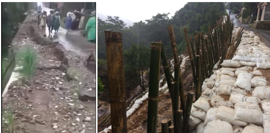
Figure 1. Before and after landslide condition
